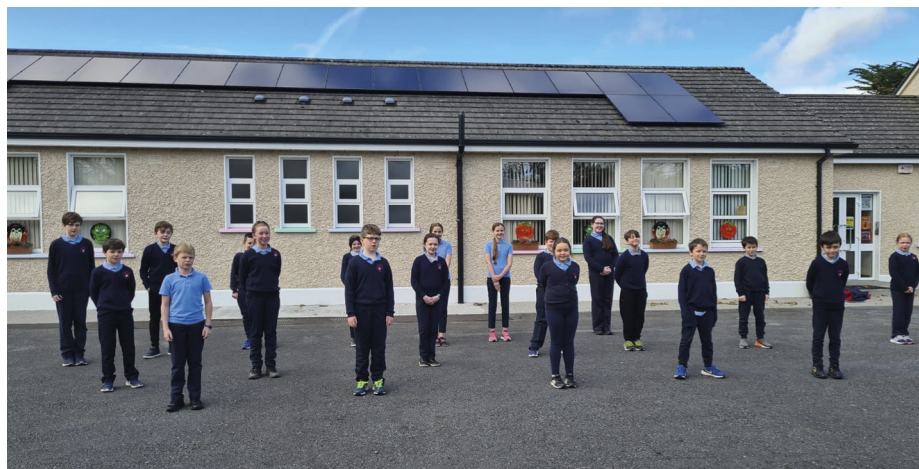
Students at St Augustine's National School, Clontuskert, Co Galway, in front of newly installed solar panels sponsored by Microsoft SSE Airtricity and Activ8.
